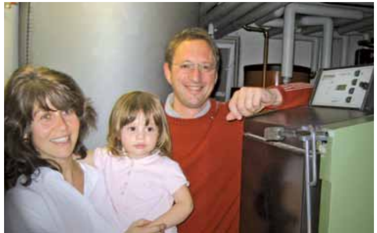
The Moser family uses an HDG Navora with 30 kW and a 2000 l accumulator for heating.
