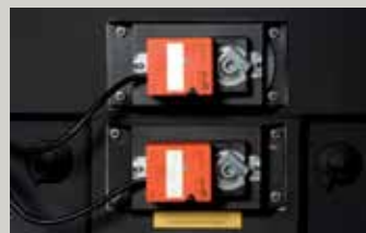
Primary and secondary air control unit
